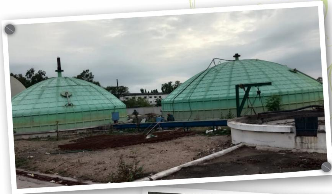
Processing plant at Waluj
