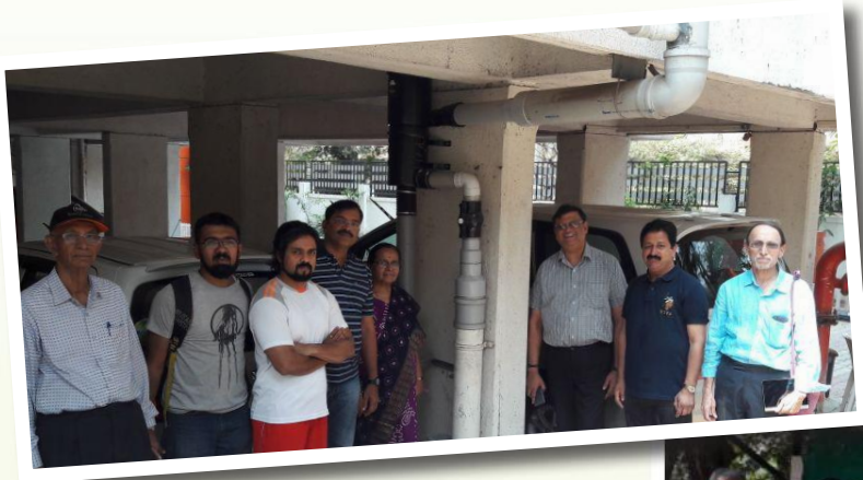
Rainwater Harvesting Unit at Laxmi Park, Navi Peth
