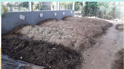
Theur Composting Plant
