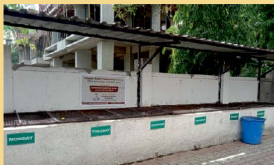
Laxmi Park Society Composting plant
